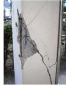
Figure 3.6. 1<sup>st</sup> storey shear cracks of column in Sendai [15].
